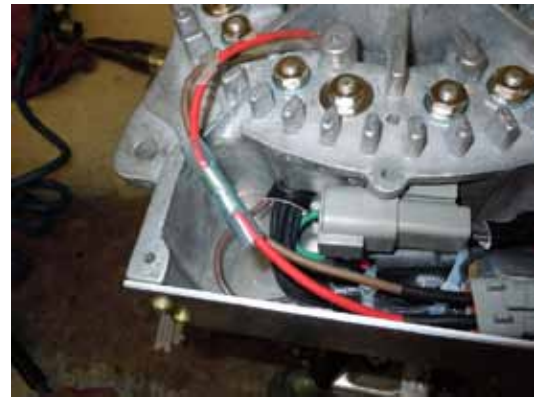
Figure 3 — Splicing to Field Coil Wires
